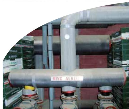
The current condition of the system shows that the insulation was able to significantly exceed 23 years of effective use. However the appearance could deceive.
